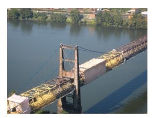
Photo taken from the hilltop on W. Va. side, showing the progress of the 2010 rehabilitation work by West Virginia DOT, taken Aug 28, 2010. Yellow paint on box truss frame visible as is the blue on the main cable. Tarps cover areas being sand blasted. Courtesy of Mrs. Donna Diserio of Follansbee, W. Va.
